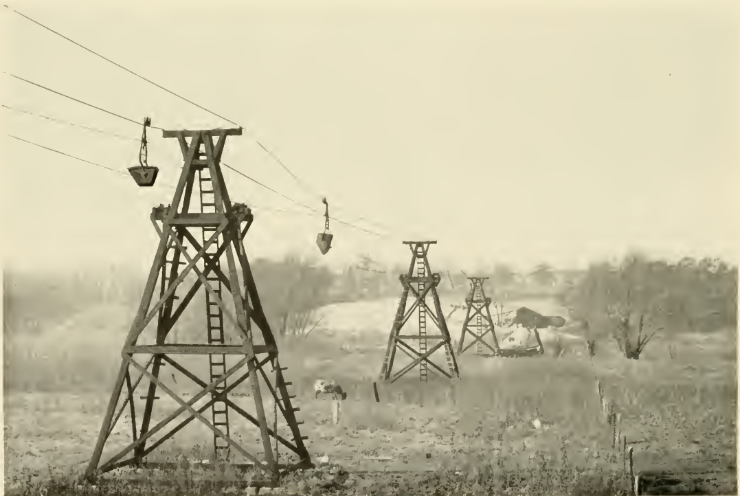
LESCHEN COMPANY'S PATENT AUTOMATIC TRAMWAY Built for Ballou's White Sand Company, Millington, Illinois
