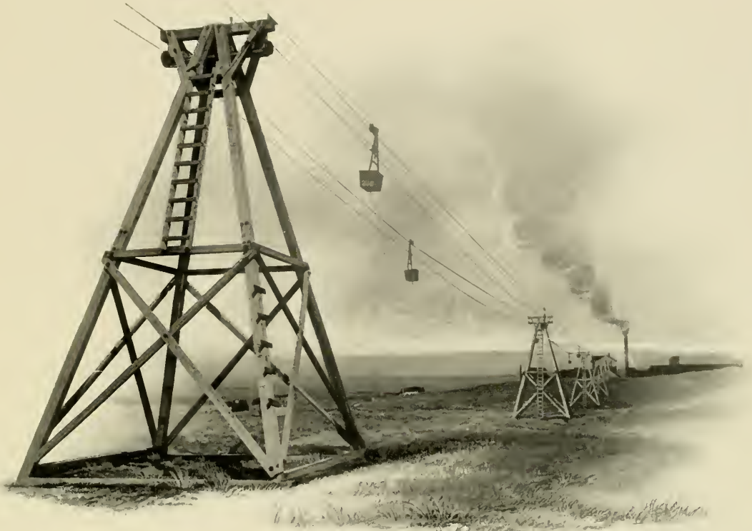
LESCHEN COMPANY'S PATENT AUTOMATIC TRAMWAY, SIXTEEN MILES LONG Built for the Penn-Wyoming Copper Company, Encampment, Wyoming
