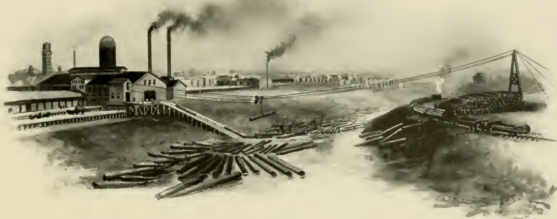
CABLEWAY HANDLING LOGS
