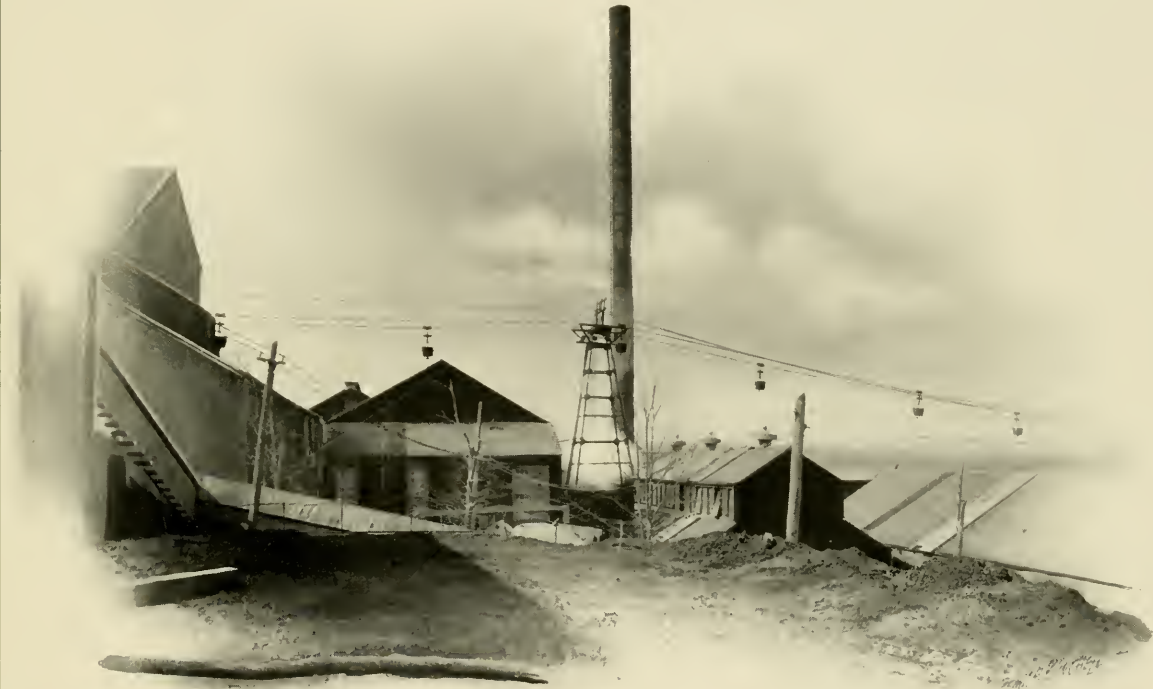
LESCHEN COMPANY'S PATENT AUTOMATIC TRAMWAY Built for Chicago Portland Cement Company, Oglesby, Illinois
