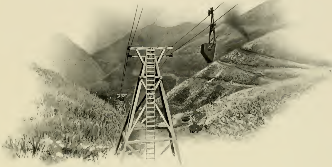
LESCHEN COMPANY'S PATENT SPECIAL AUTOMATIC TRAMWAY Built for Bingham-New Haven Copper and Gold Mining Company, Bingham, Utah
