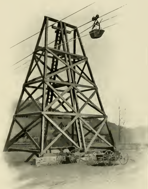
LESCHEN COMPANY'S TWO-BUCKET TRAMWAY Built for Victor Fuel Company, Hastings, Col.
