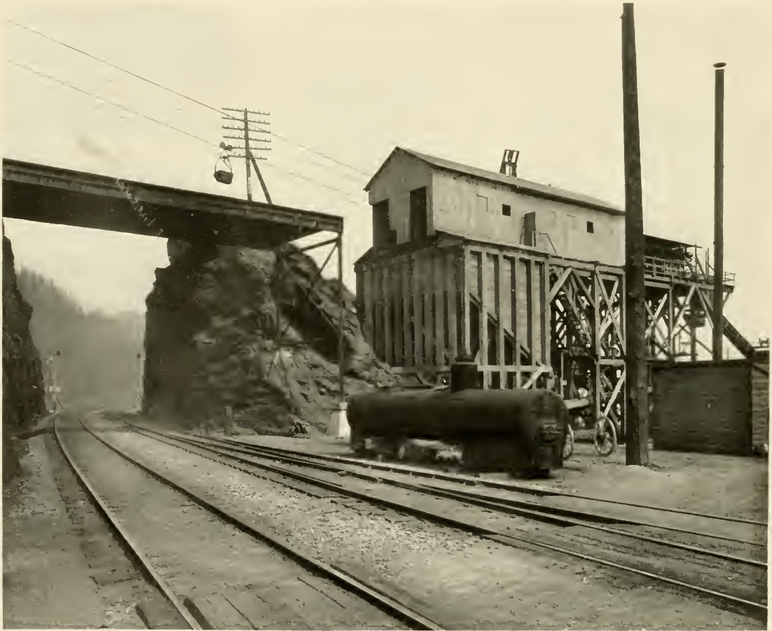
LESCHEN COMPANY'S PATENT SPECIAL AUTOMATIC TRAMWAY Built for Hudson Iron Company, Fort Montgomery, New York
