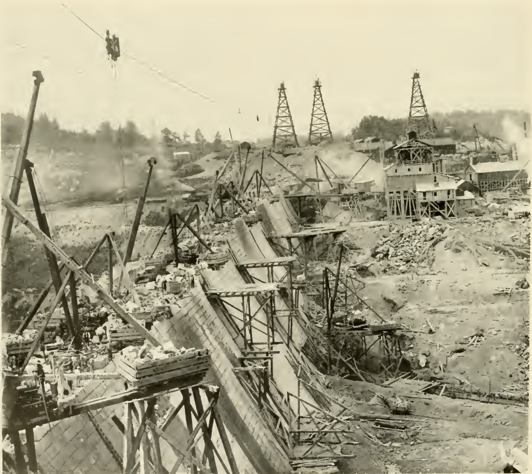
CABLEWAY USED IN THE BUILDING OF DAM
